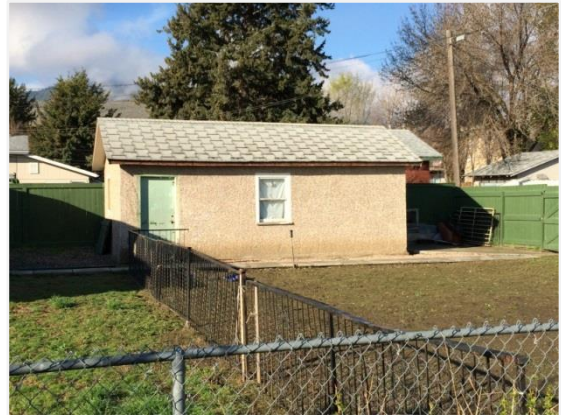
Example of a typical residential area accessory building
